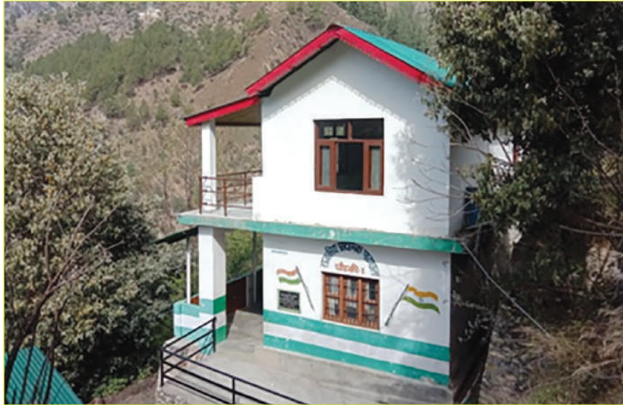
Construction of 2 rooms of Govt. Primary School, Chowki
