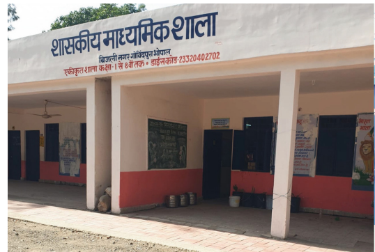
Image 9: Govt. Primary School, Govindpura
