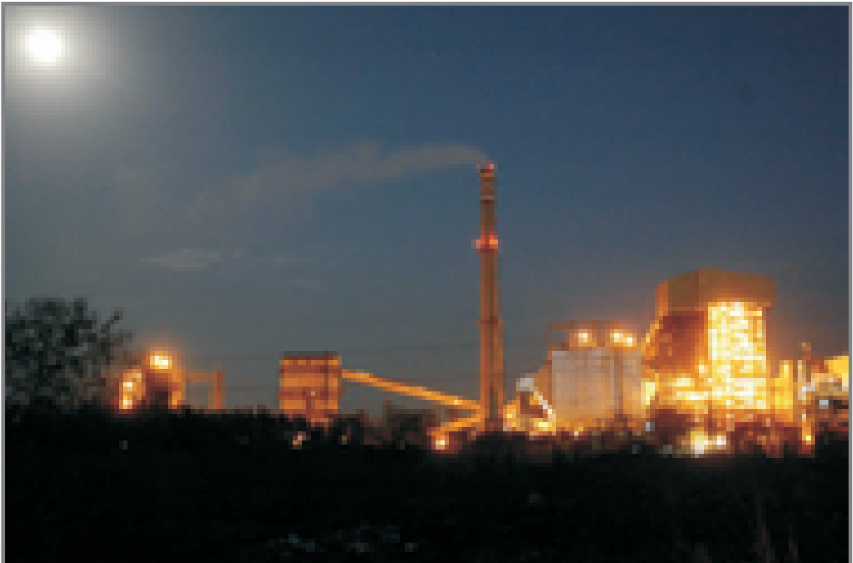
HEG's captive power plants meet more than 90 per cent of its power requirements.
